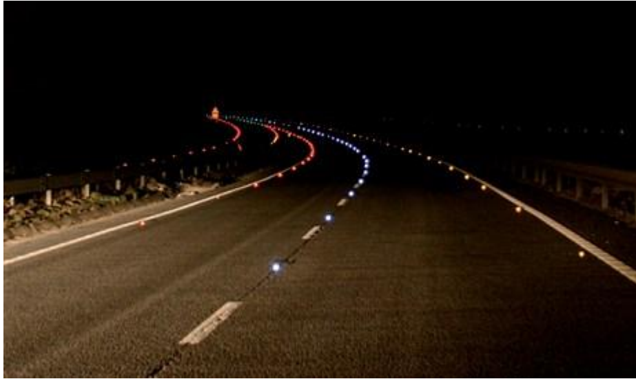
Figure 1: Astucia SolarLite Intelligent road studs have safely guided vehicles to the English port of Dover (World Highways, 2010)
